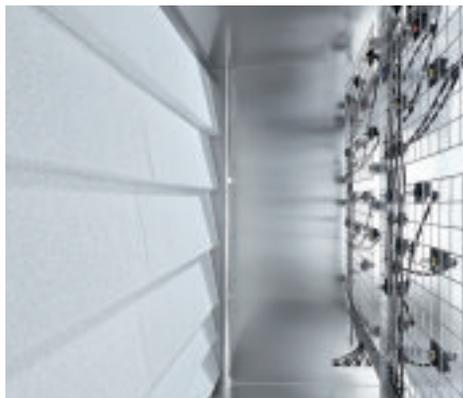
The Condair DL is a hybrid humidifier that combines spray and evaporative technologies to maximise moisture absorption and provide humidity control at  $\pm 2\%RH$ . A water treatment system provides pure water to a grid of nozzles located inside the duct.
